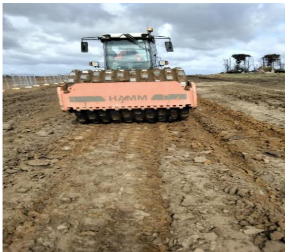
Photograph 3: Proof roll with Pad foot
