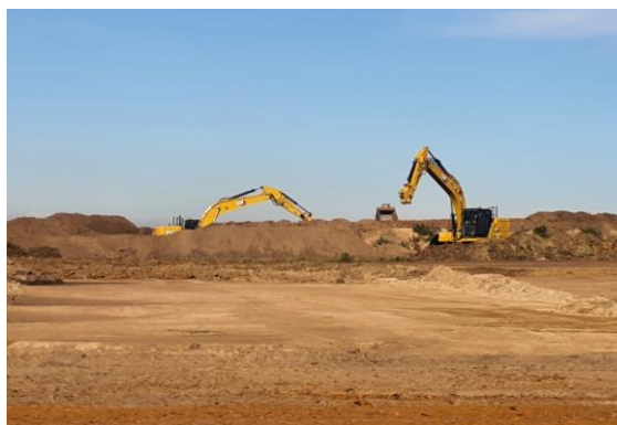
Photograph 6: Excavator placing fill
