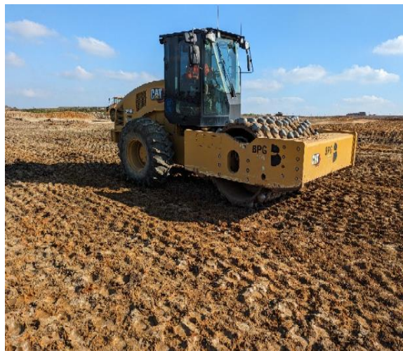
Photograph 4: Subgrade assessment with 15 Tonne Pad foot Roller
