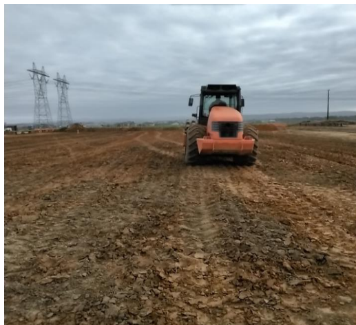
Photograph 6: Pad foot compacting clay
