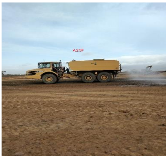
Photograph 7: Water cart used for moisture conditioning
