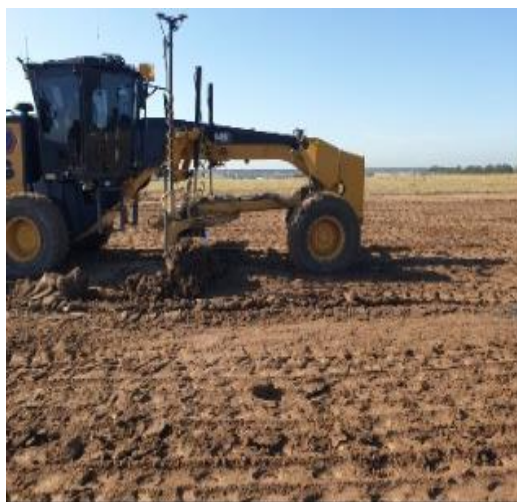
Photograph 8: Grader spreading material
