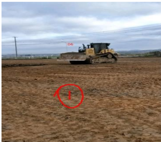
Photograph 5: D6 Dozer used during filling.
