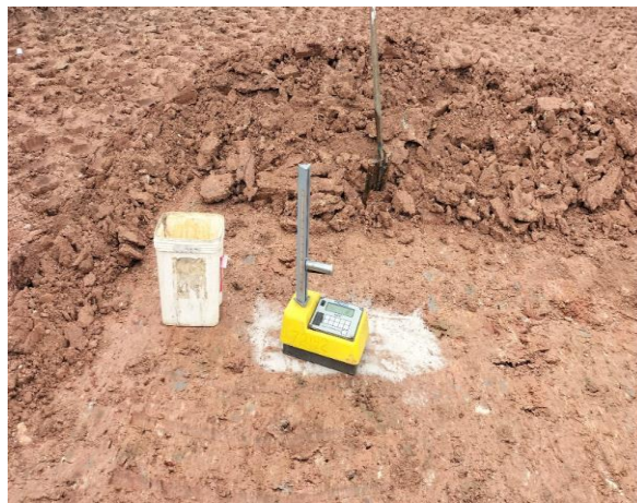
Photo 10: Field density/moisture test
