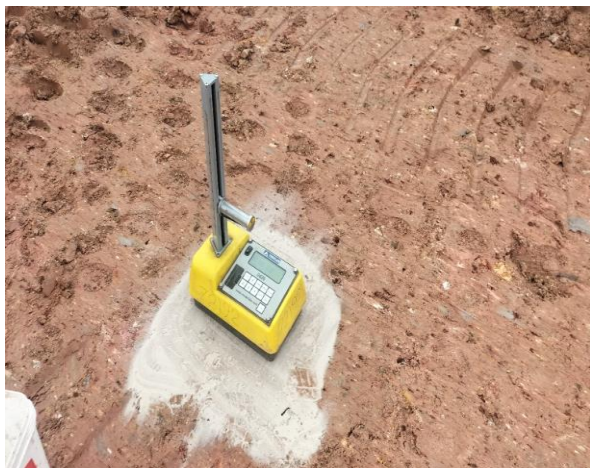
Photo 9: Field density/moisture test
