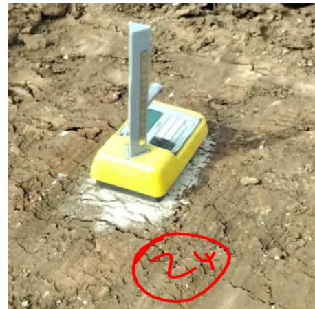
Photo 10: Density Test with sand
