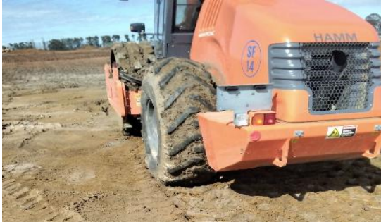
Photograph 2.7.1: Material Compaction
