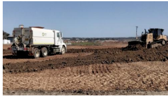
Photograph 2.2: Moisture Conditioning, September 2021
