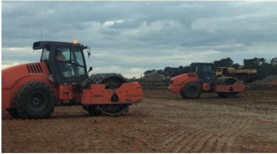
Photograph 2.1: Material Compaction, August 2021
