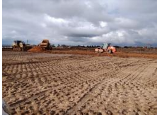
Photograph 2.2: Material Delivery, August 2021
