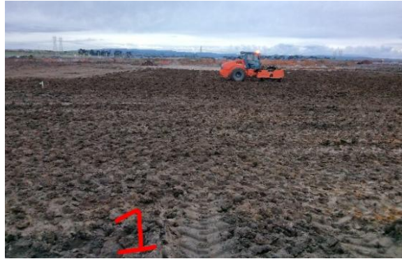
Photograph 2.2: Material Compaction, June 2021
