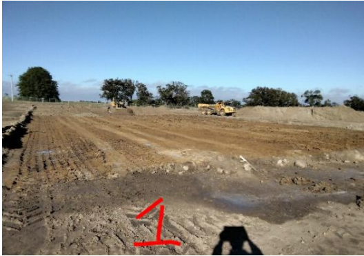
Photograph 2.1: Material Delivery, May 2021
