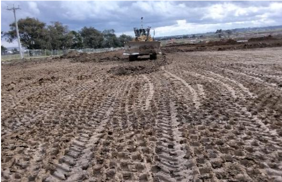
Photograph 2.1: Earthwork operations, June 2021
